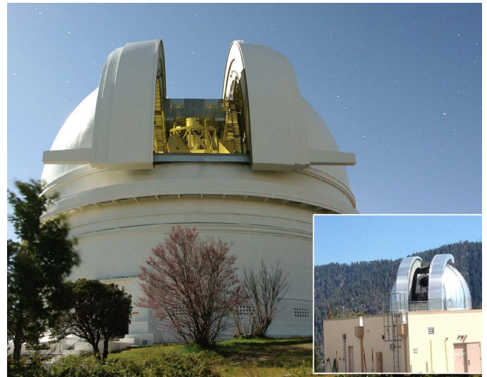
Palomar Observatory's Hale Telescope will receive the high-rate data downlink from the DSOC flight transceiver. Inset: A high-power near-infrared laser transmitter at JPL's Table Mountain facility, shown, will transmit low-rate data to the transceiver. Credit: NASA/JPL-Caltech/Palomar Observatory
